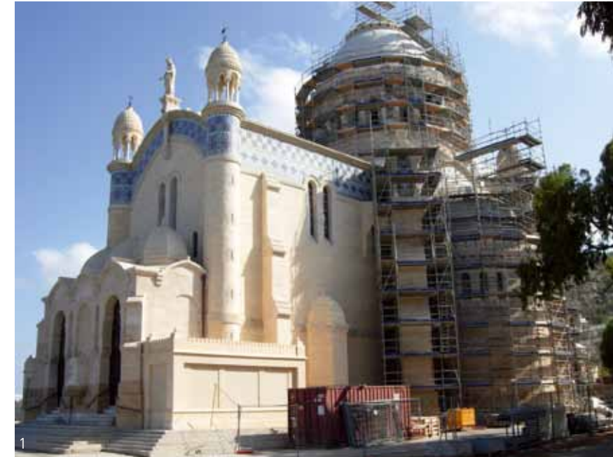
1. Our Lady of Africa - restoration works in progress
